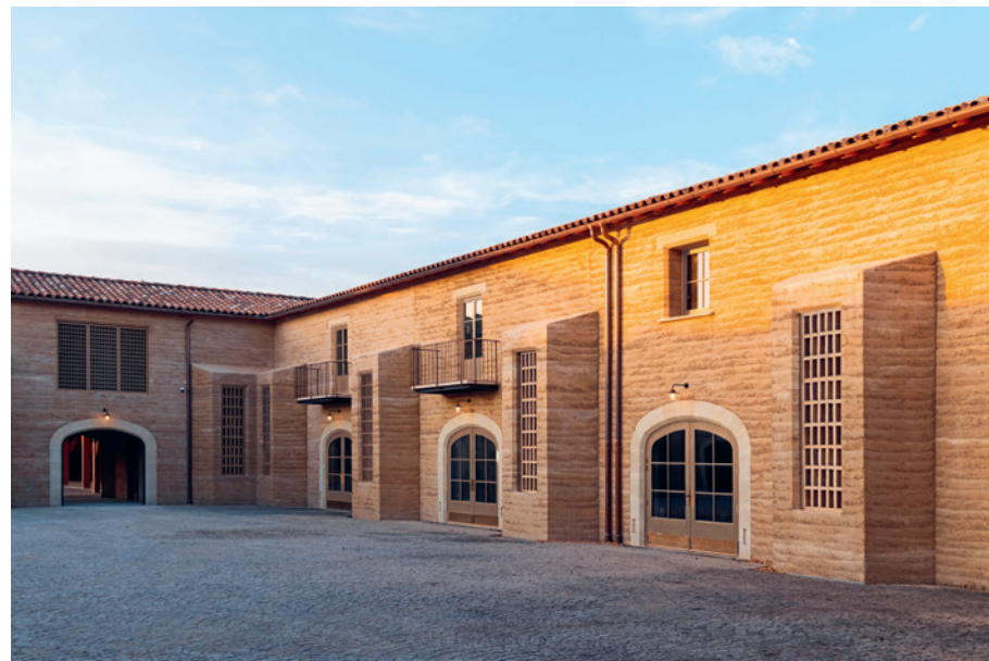
Innenhof schützt vor Mistral und dient zur Lüftung. Interior courtyard provides protection against the mistral and serves as ventilation.
